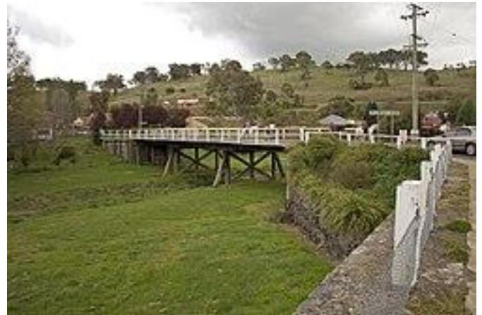
Belubula River Bridge in Carcoar NSW
